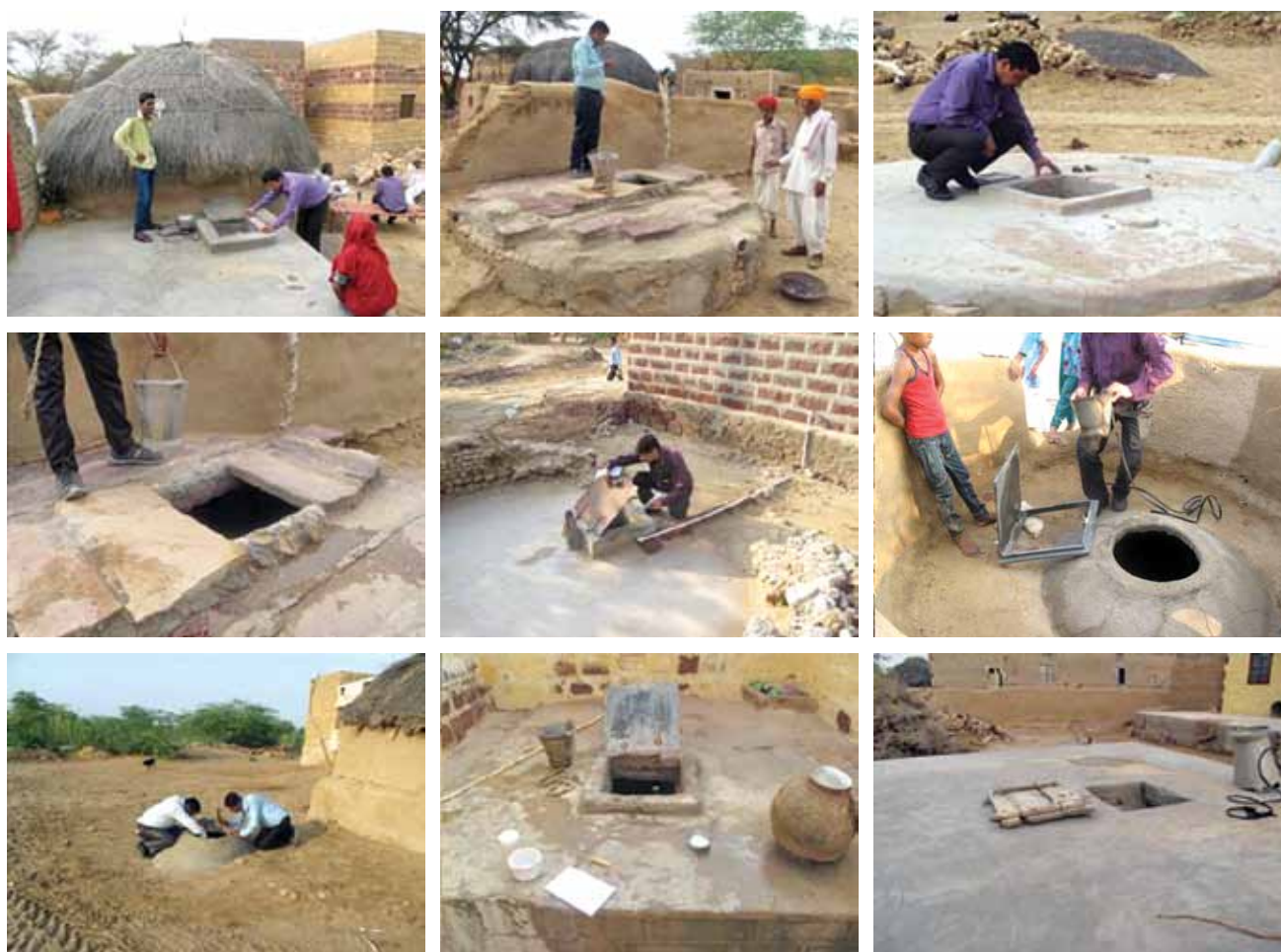
Fig.15: Evaluation and marking of lids for replacement.
